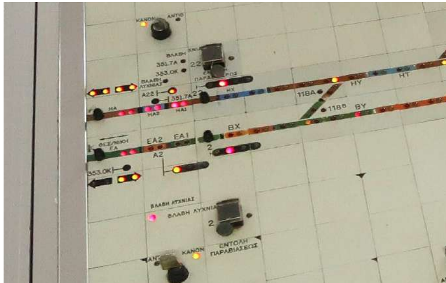
Figure 49. Section EA3 (indicated EA to the left of EA2 on the picture) of the control panel incorrectly indicating an occupation.
