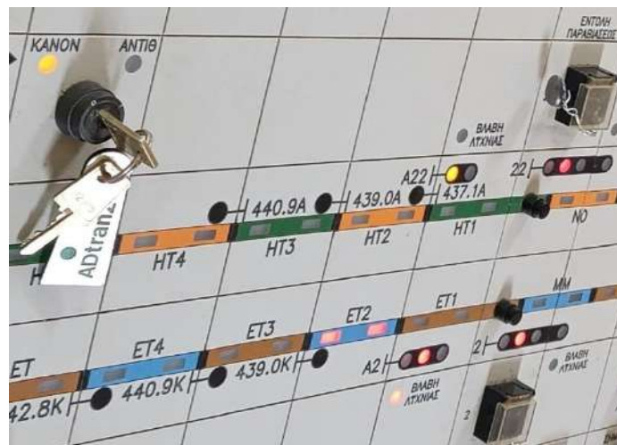
Figure 39. Position and movement of trains, here in the section ET2 depicted on Katerini Station control panel.
